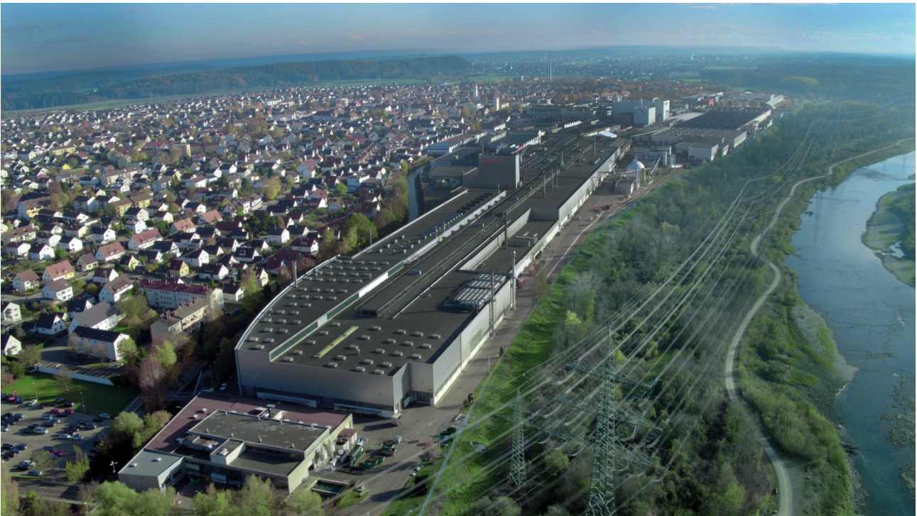
Wieland's production site in Vöhringen (Germany) - Photo courtesy of Wieland Group
