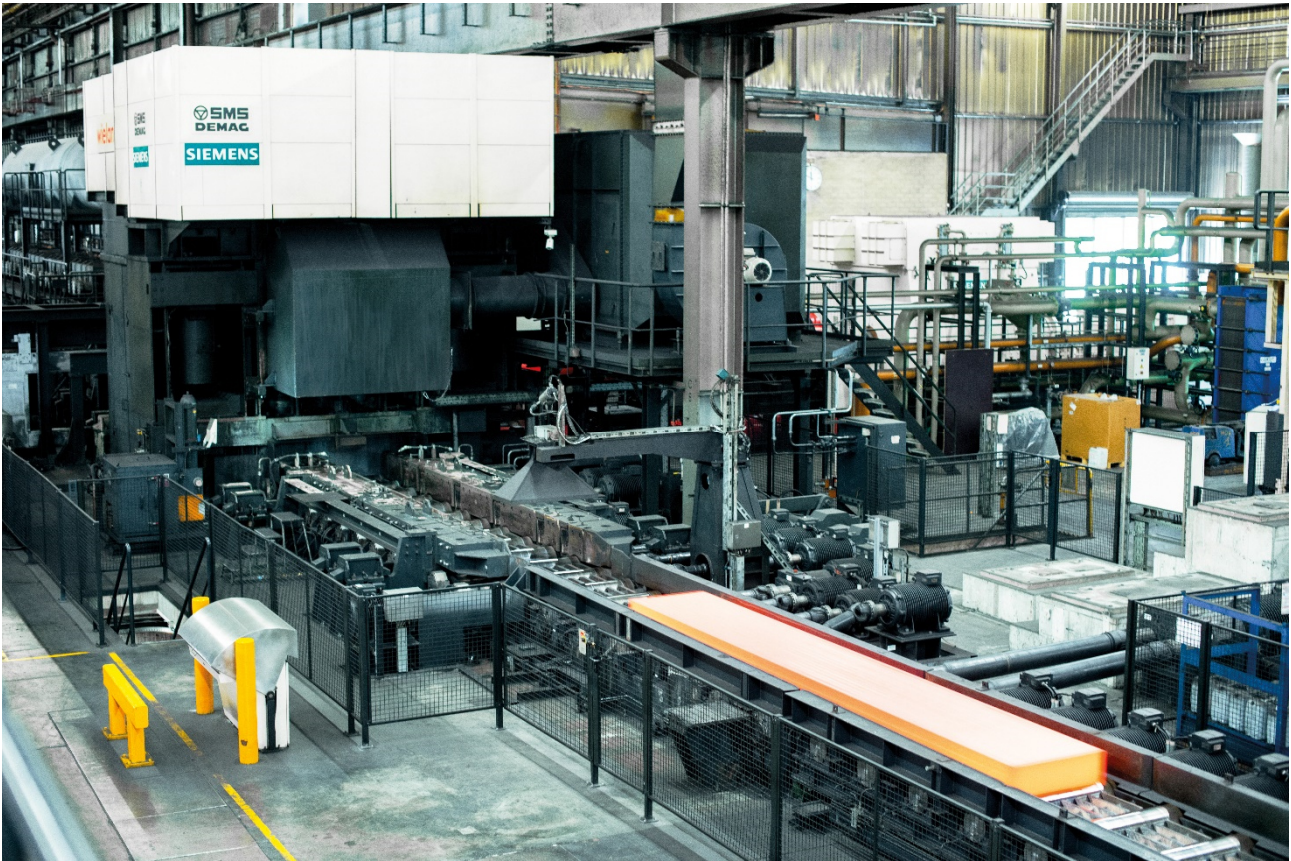
Hot rolling mill at Wieland's plant in Vöhringen (Germany) - Photo courtesy of Wieland Group
