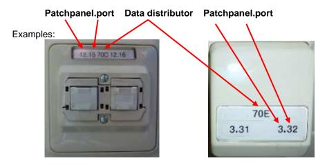
2.4.2 For connections via the structured Ethernet cabling that are documented not only by IT but are also managed e.g. in a system documentation, and can only be identified there by a special device identifier, a plant device identifier is added to the IT device identifier.
