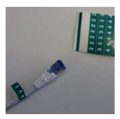
Patch cables that leave the data distributor (exceptional case) receive a device identifier like a simplex cable.
