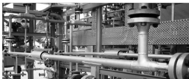
Fig. 2 Photo of Fouling Test Section.
