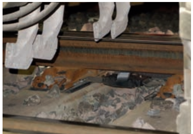
Tamping with installed Austroroll rollers.
