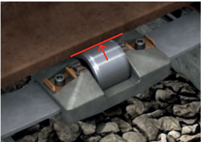
The roller in contact with the switch blade before rolling up, with horizontal force component.
