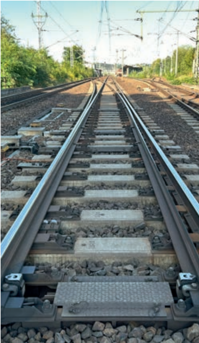
Austroroll in a new constructed EW UIC60-760-1:14-w with hollow sleeper.
