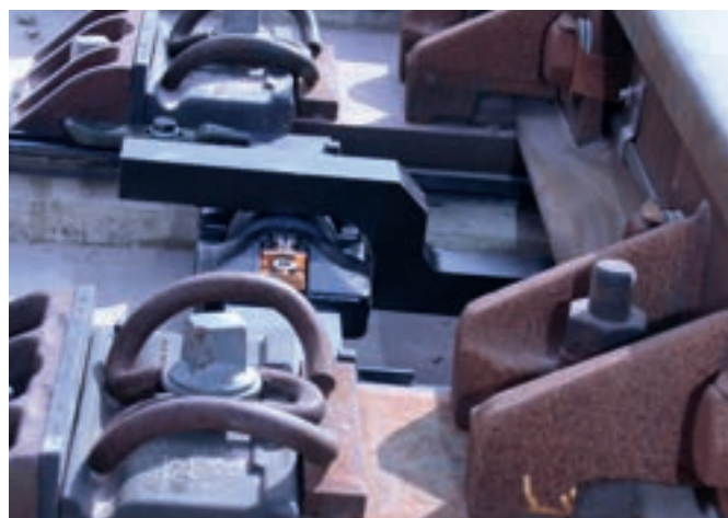
Austroroll MFR on slab track, type W300.
