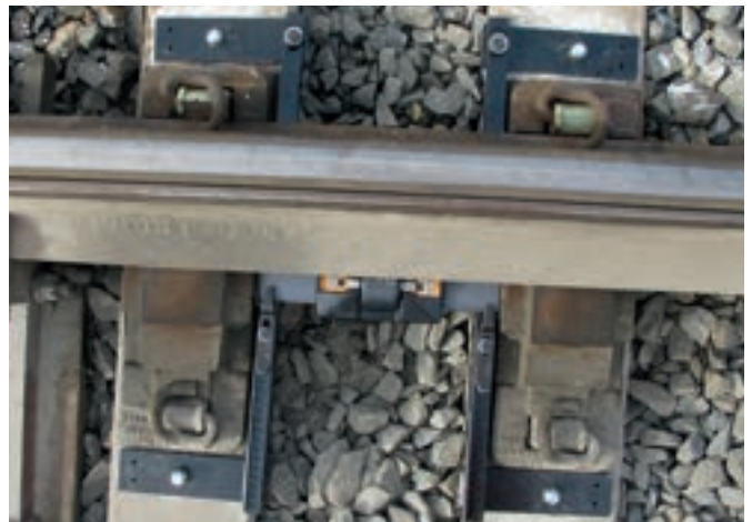
Special design using composite anchors on concrete sleepers.
