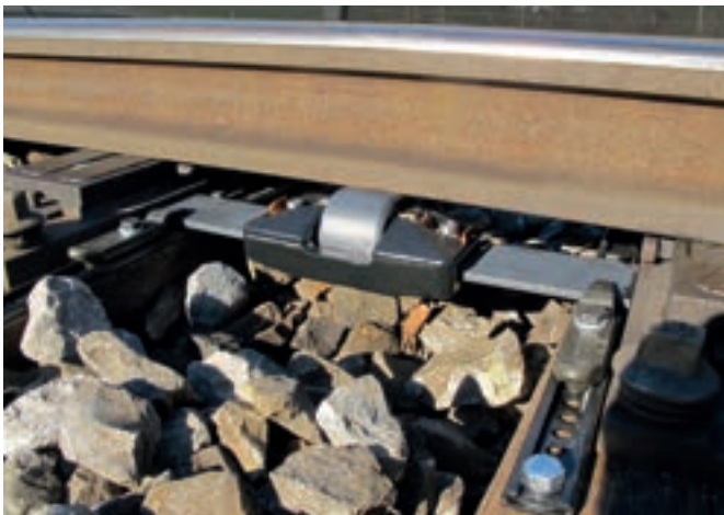
Austroroll with direct mountings on wooden sleepers.
