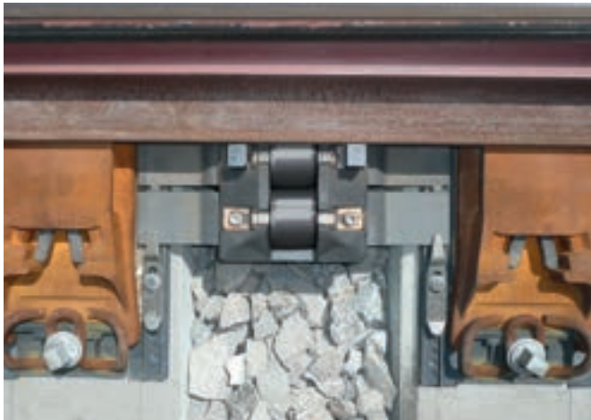
Double roller in "new construction version" with mounting plates in an EW UIC60-1200-1:18.5-w-VS.
