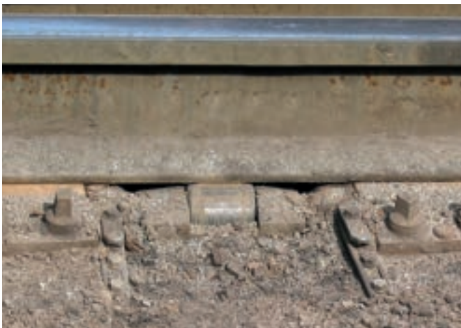
Austroroll under extreme conditions in a steelplant steelwork.
