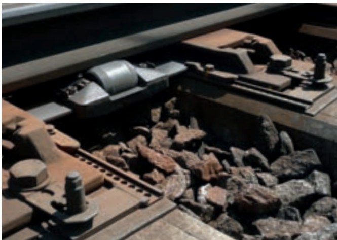
Austroroll in a retrofit version for a switch point on concrete sleepers.
