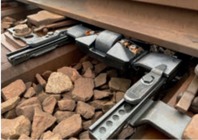
Retrofitting of turnouts with BWG slide chairs.
