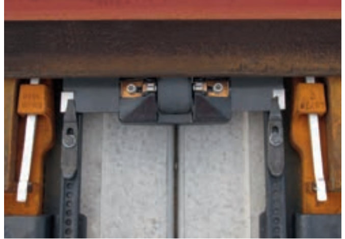
Austroroll in a high speed line with slab track.
