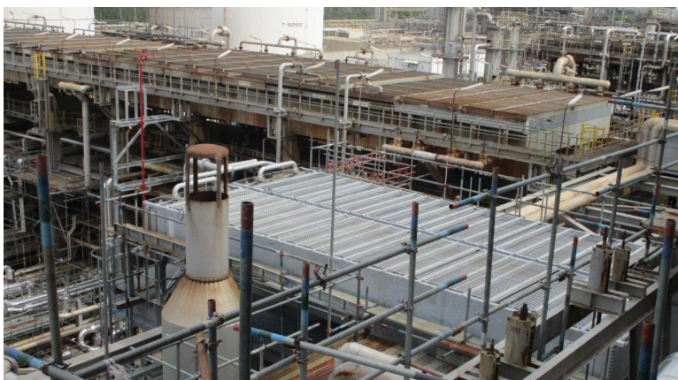
Figure 11. VGO cooler equipped with DIESTA tubes.
