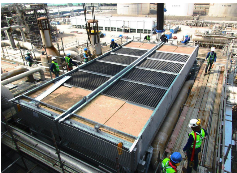
Figure 10. DIESTA bundle installation with typical plywood protection plates.
