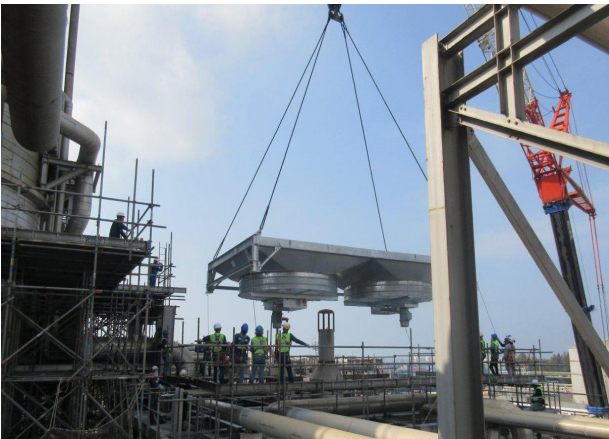
Figure 9. Erection of the lower part on the pipe rack.
