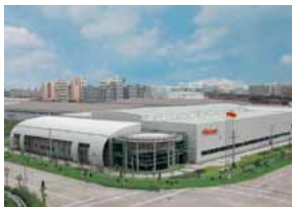
Wieland Metals Shanghai Limited, Shanghai, China
