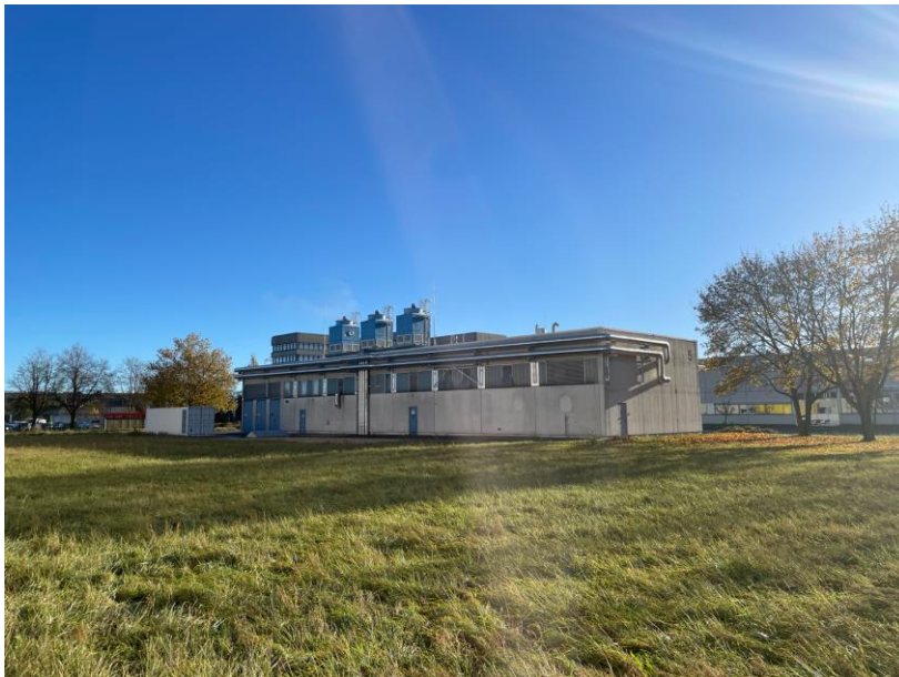
Exterior view of Wieland Group's modernized heating system in Ulm.
